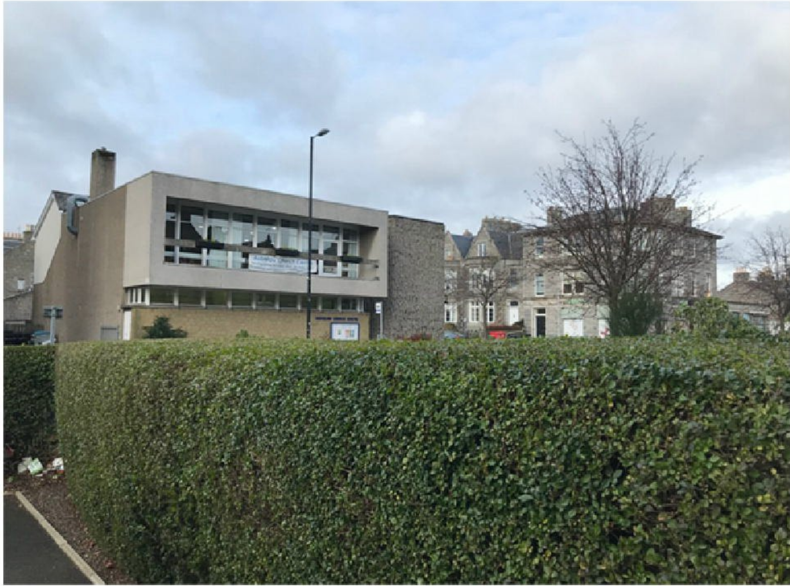
Photo 09. Rubislaw Church Centre taken from front door of 18 Fountainhall Rd
